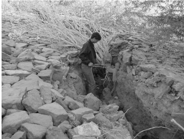
Figure 5. Open Fissures on the upstream face of Fatehgadh Dam (courtesy EERI 2001)
