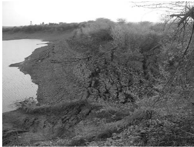
Figure 3. Failed upstream slope of Chang Dam (courtesy EERI 2001)
